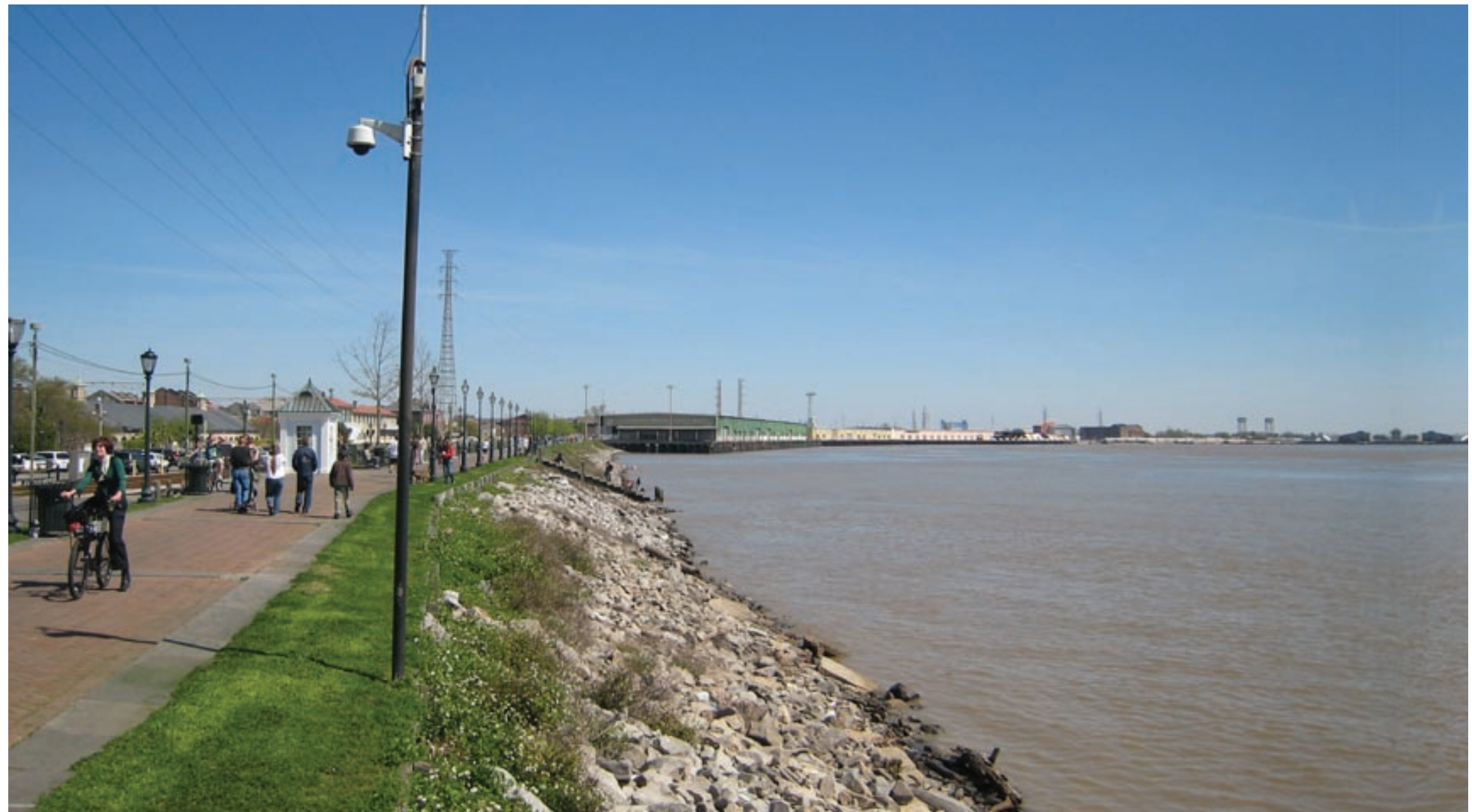
Existing Conditions of Levee and Pedestrian Walkway at Moonwalk
