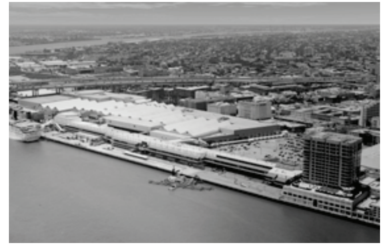
Existing Conditions at Julia Street
