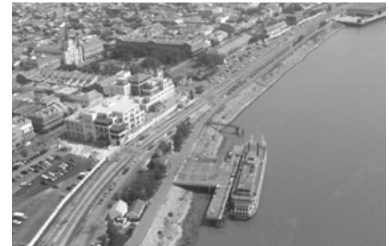
Existing Conditions at Moonwalk
