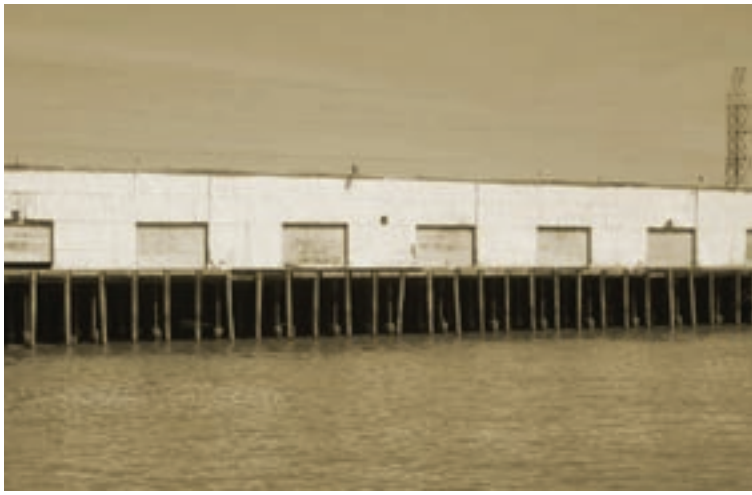
View of Existing Mandeville Wharf Looking from Mississippi River
