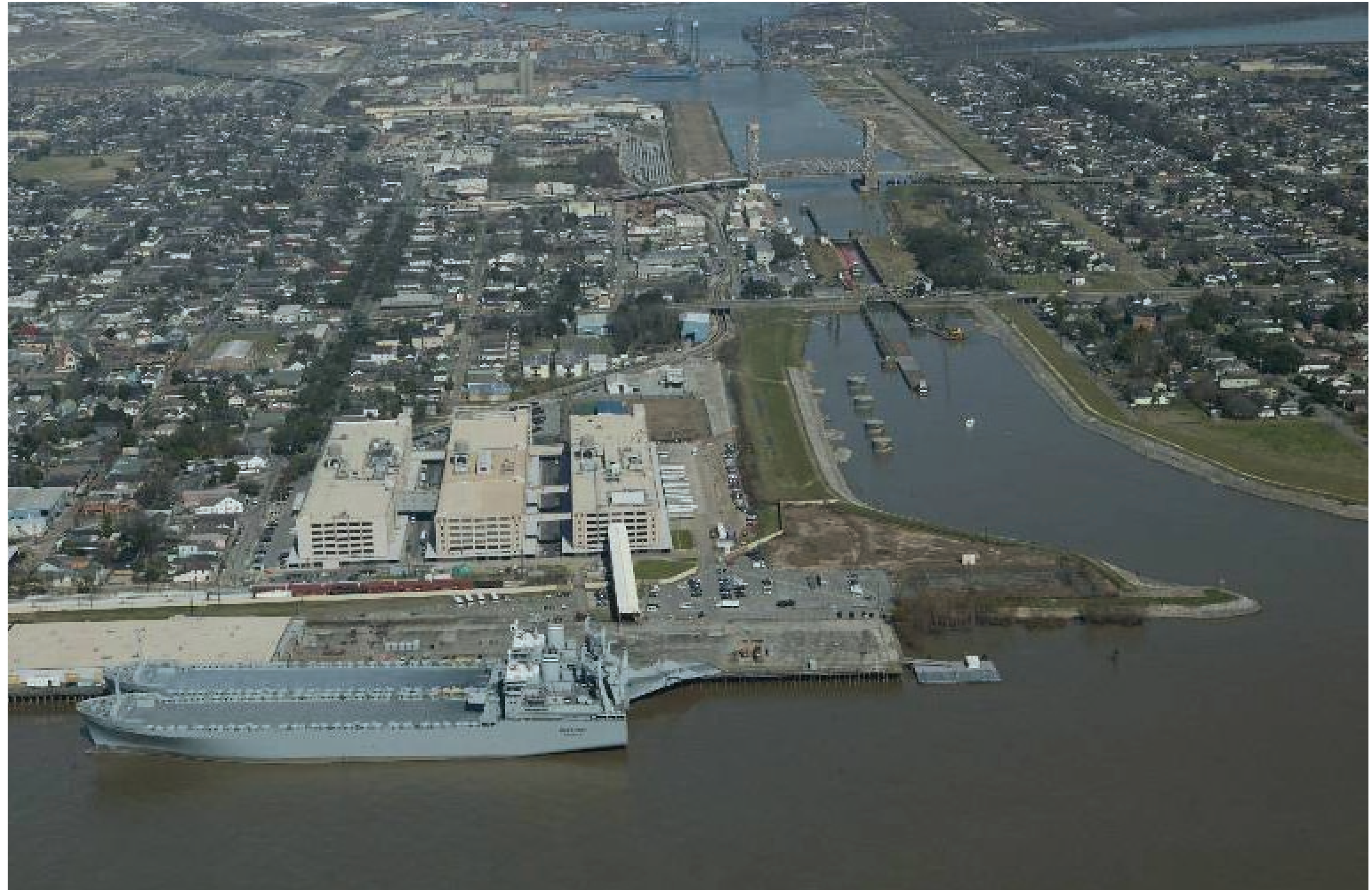
View of Existing Department of Defense Complex at Poland Avenue, Industrial Canal and Mississippi River
